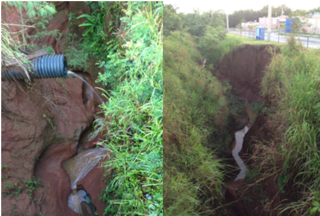
Figure 10. Extensive gully erosion causing sediment transport and infrastructure risk (#7)
