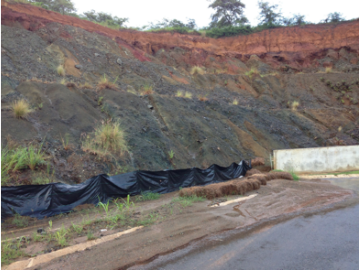
Figure 6. Extensive gully erosion and sediment transport from the hillside (Project #5)
