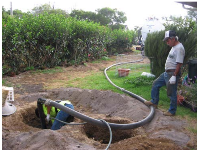
Pumping Septic Tank
