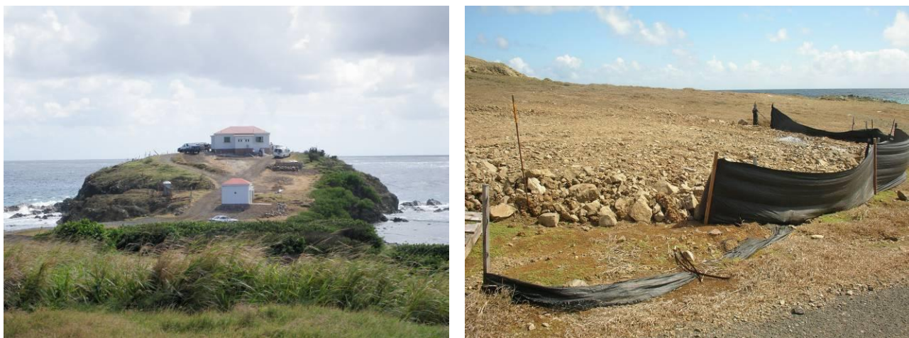
Figure 7.3. Residential construction (left) and ESC practices (right) on Grass Point associated with the Pt. Elizabeth development.
