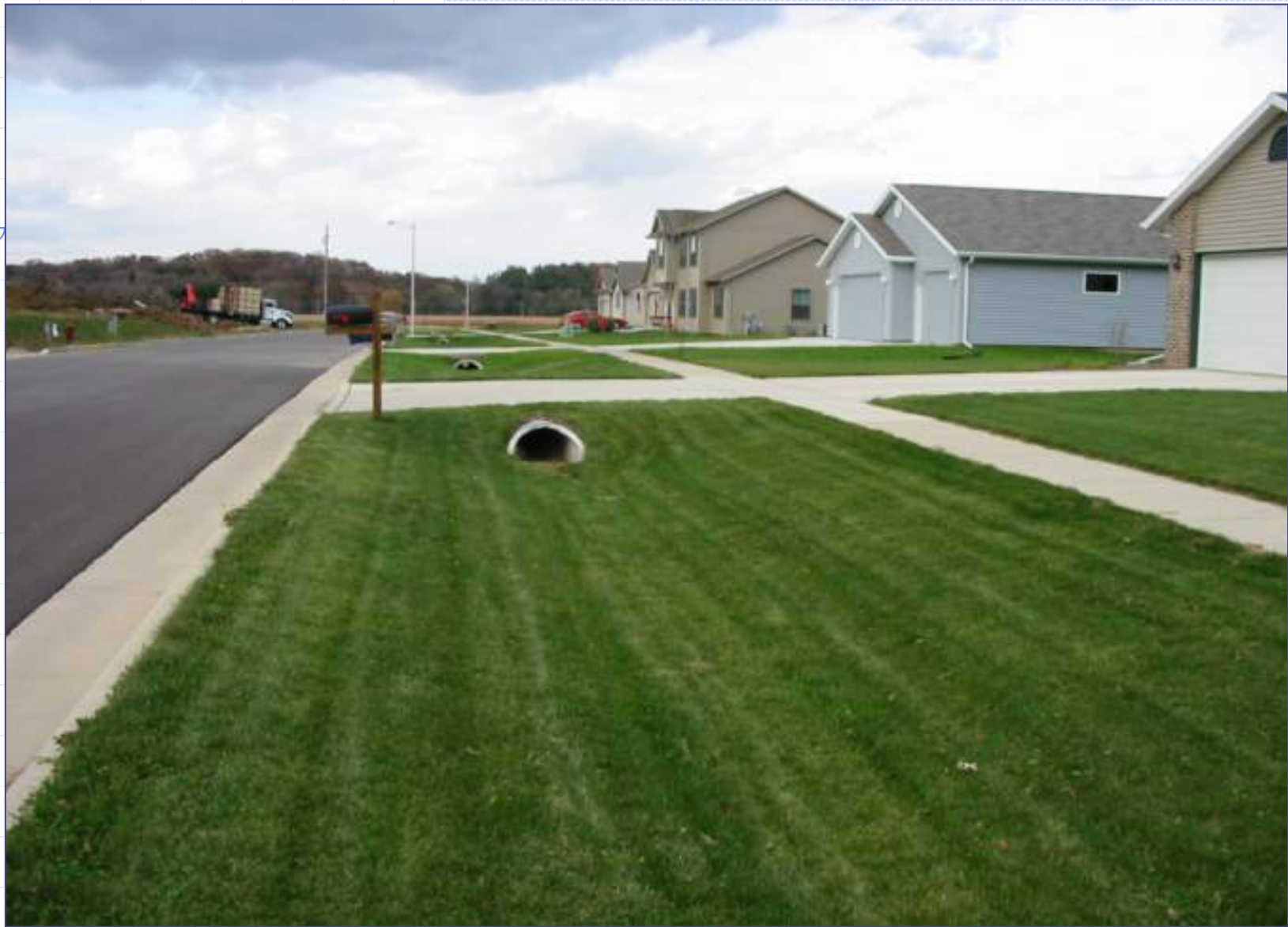
Nominee No. 1: The high input swale with curb
