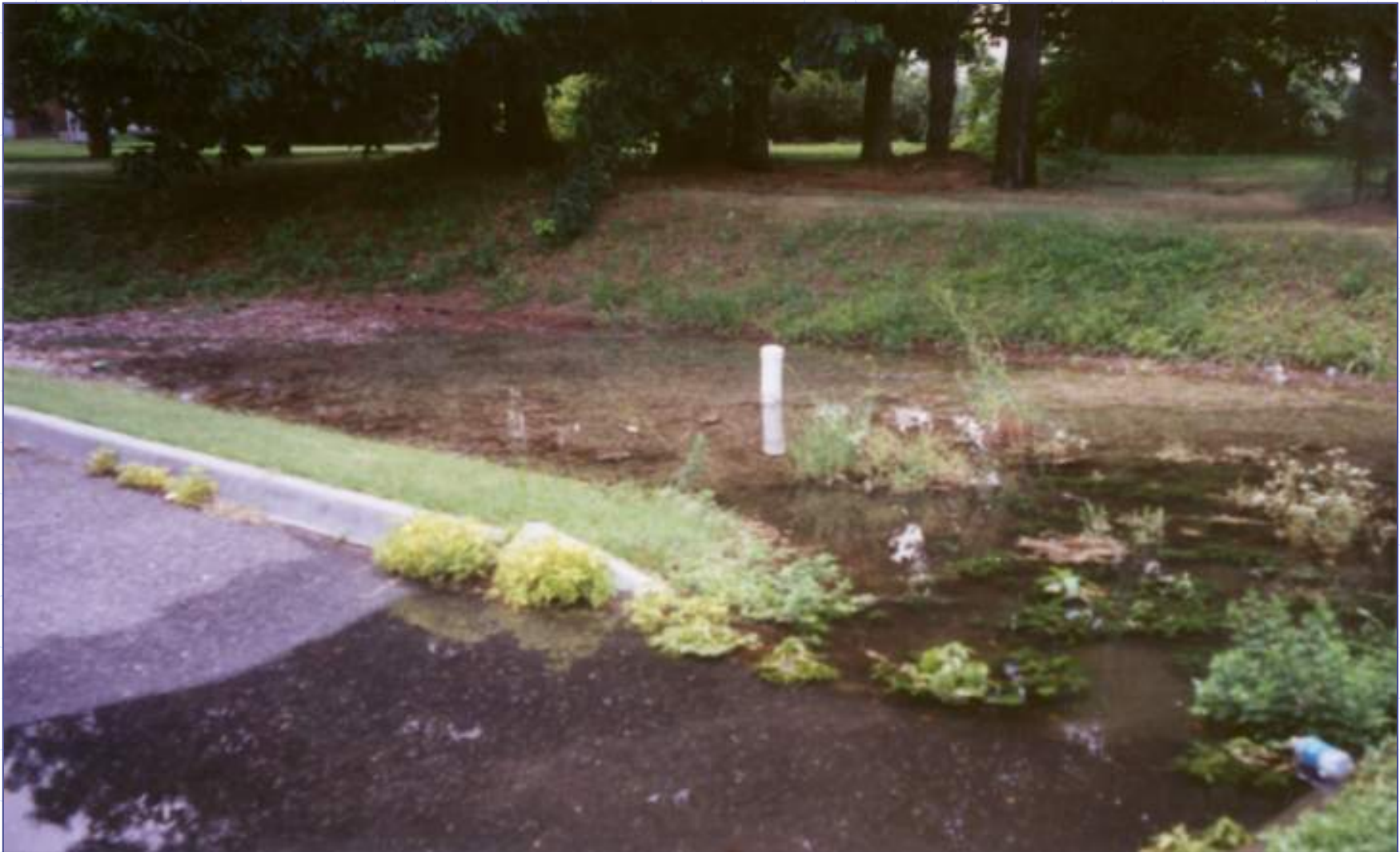
Nominee No. 2: The infiltration trench that couldn't
