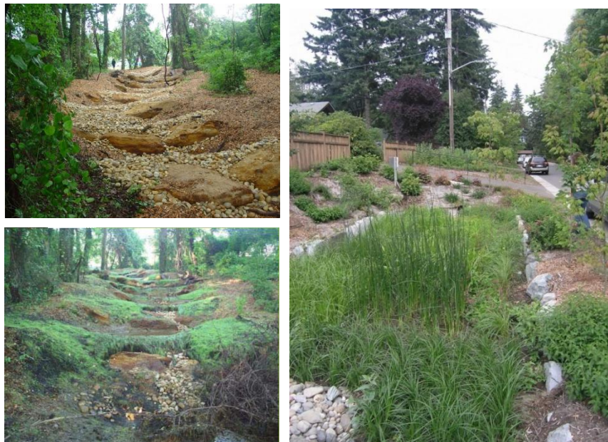
Figure 12. Photos showing stepped conveyance systems in channel from Anne Arundel County, MD (two photos on left), and a linear bioretention facility along a residential street in Seattle, WA (on right)
