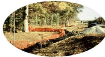
5. Erosion & Sediment Control
