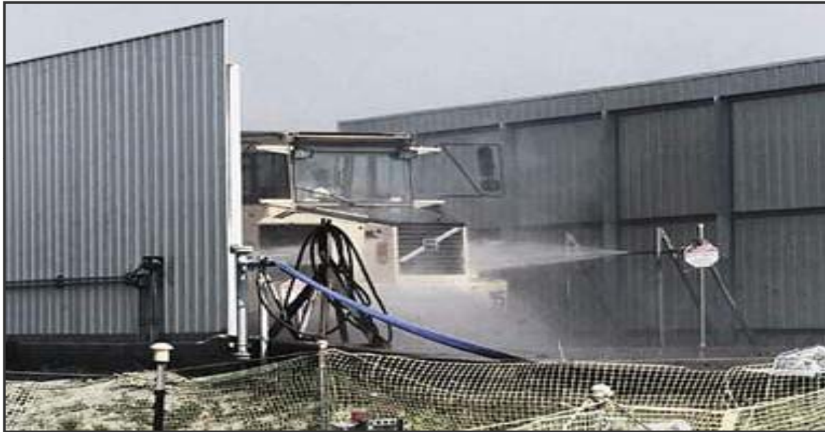
Dedicated truck wash site with runoff controls (Source: US DOE)
