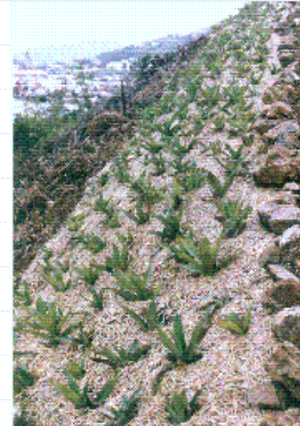
Hydroseeding used to control erosion on slopes during earth change operations.
