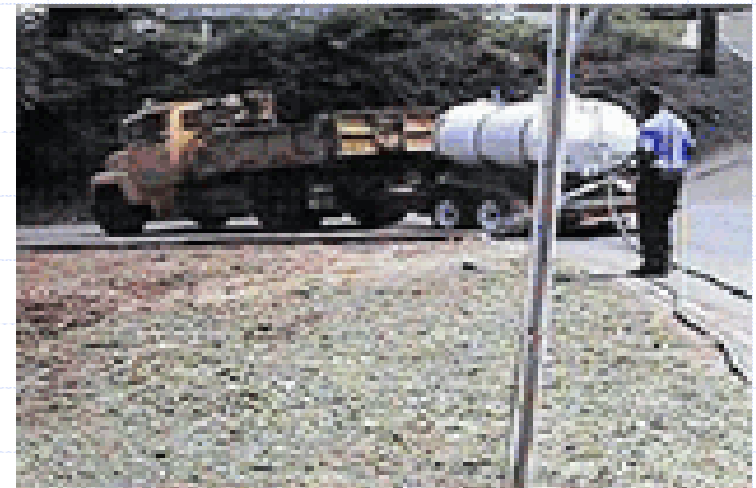
Hydroseeding used to control erosion on slopes during earth change operations.
