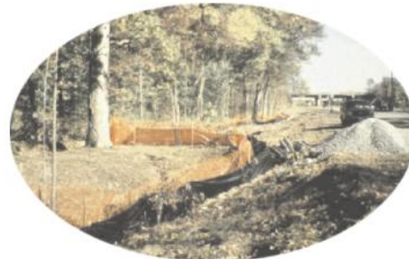
5. Erosion & Sediment Control
