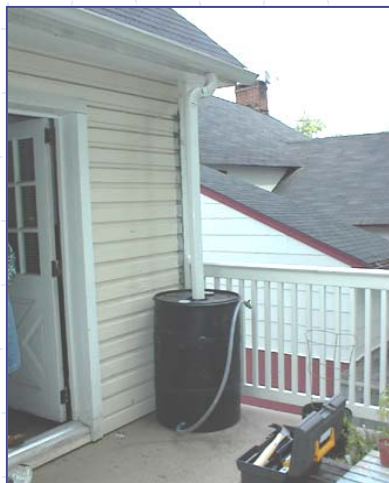
Disconnected; Flowing to Rain Barrel
