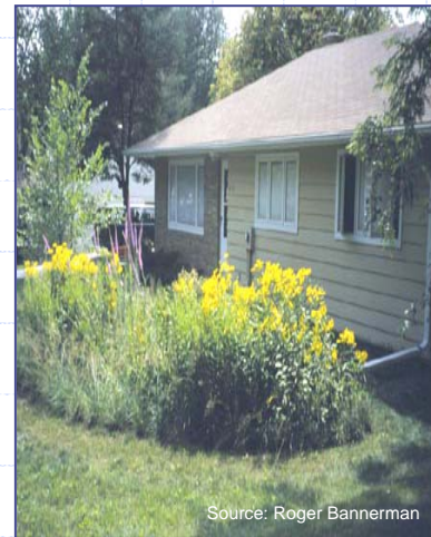
Disconnected; Flowing to Rain Garden
