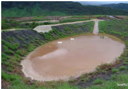
Newly constructed storm water pond at landfill
