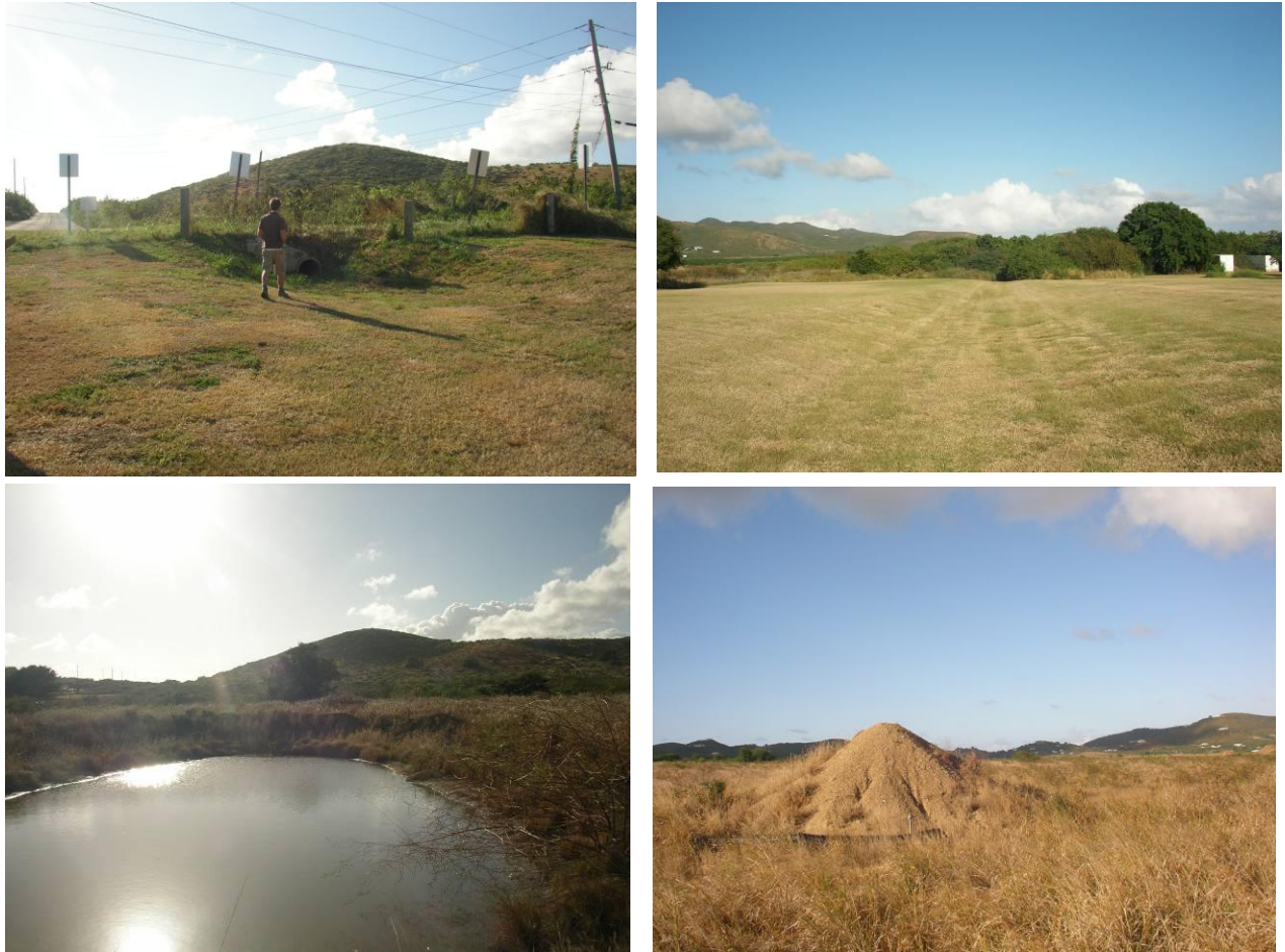
Figure 8.9. Clockwise from top left: Culvert leading from Southside Rd. to grass swale at Boy Scouts site; Grass swale leading from culvert outfall to Great Pond on Boy Scouts property; Detention pond adjacent to Great Pond near Boy Scouts property; Soil mounds from Wyndham excavation.
