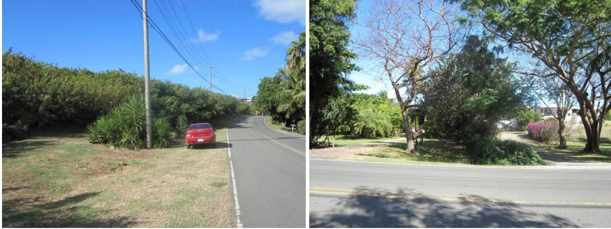
Figure 4.32. Runoff from the East End Rd. flows into the grassy depression along the south side of the road (left) as well as the swale and depression between and to the left of the driveways, respectively (right).
