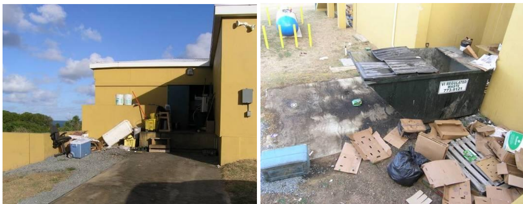
Figure 4.10. Blue Water Terrace has an uncovered area where cleaning products appear to be rinsed (left) and an uncovered dumpster/materials storage area with evident leaking and staining (right).
