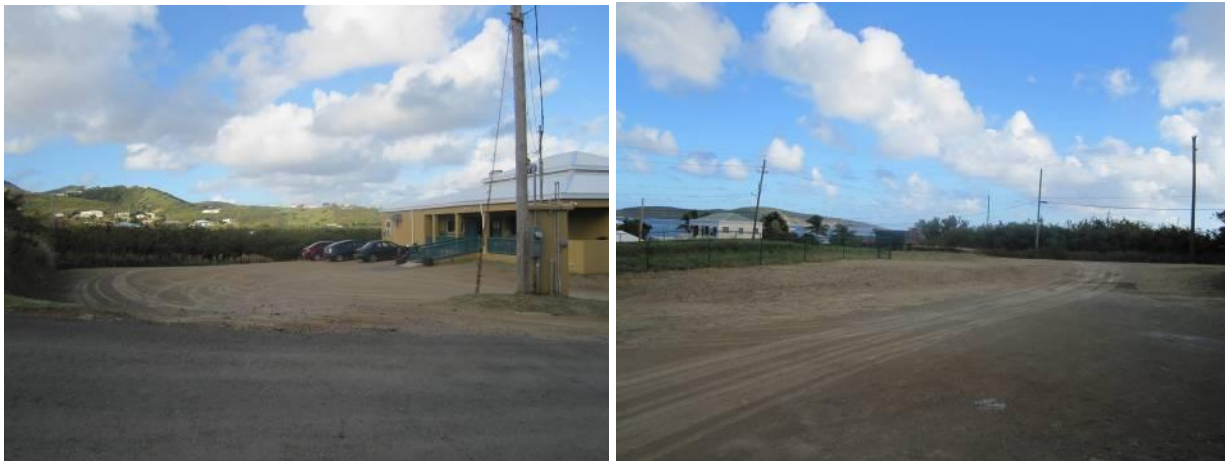
Figure 4.11. The grassy area in the far left of this photograph is a good location for a bioretention facility for runoff from the parking area (left). This depression on the north side of the building could also be converted to manage stormwater from the property (right).
