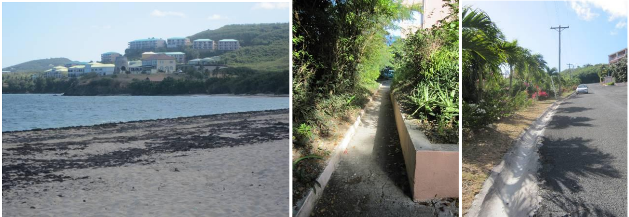
Figure 4.16. Coakley Bay condos are located on a steep hillside overlooking Coakley Bay (left). Stormwater is conveyed through the site via paved swales (middle and right).
