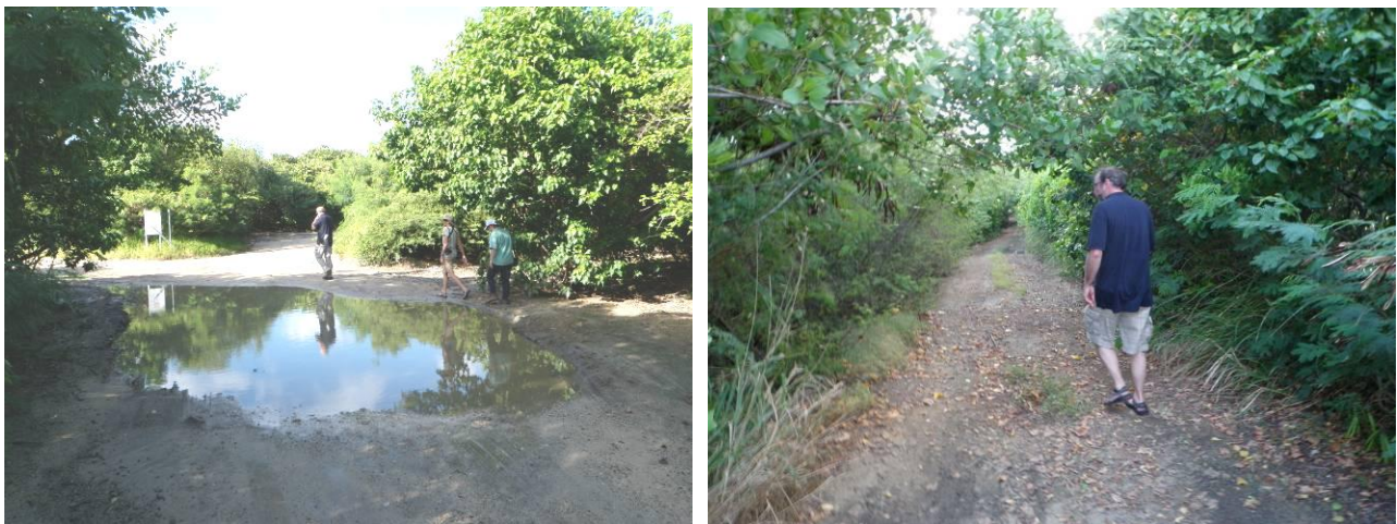
Figure 3.4. Standing water in the current road/parking area (left); the embankment (right).
