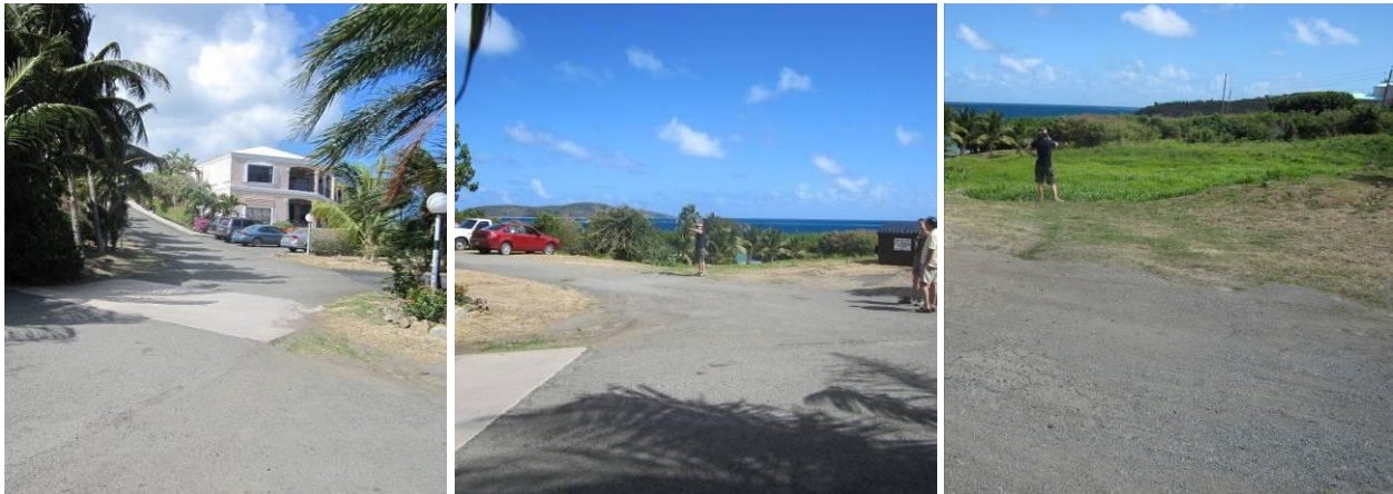
Figure 4.20. Stormwater runoff is conveyed across the entrance road with a shallow water bar (left) and continues towards the parking area near the dumpster (middle), eventually, flowing down into a grassy depression that exists in an undeveloped lot (right).
