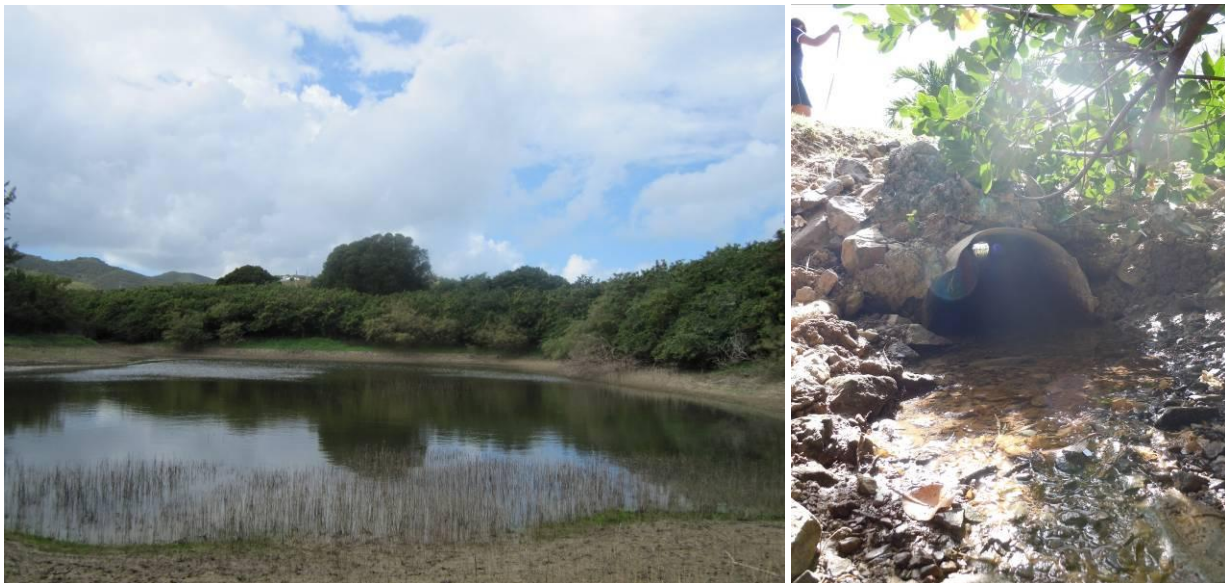
Figure 4.1. Pond along gut in Cotton Valley Neighborhood (left) and culvert at East End Road discharge location to Yellowcliff Bay (right).
