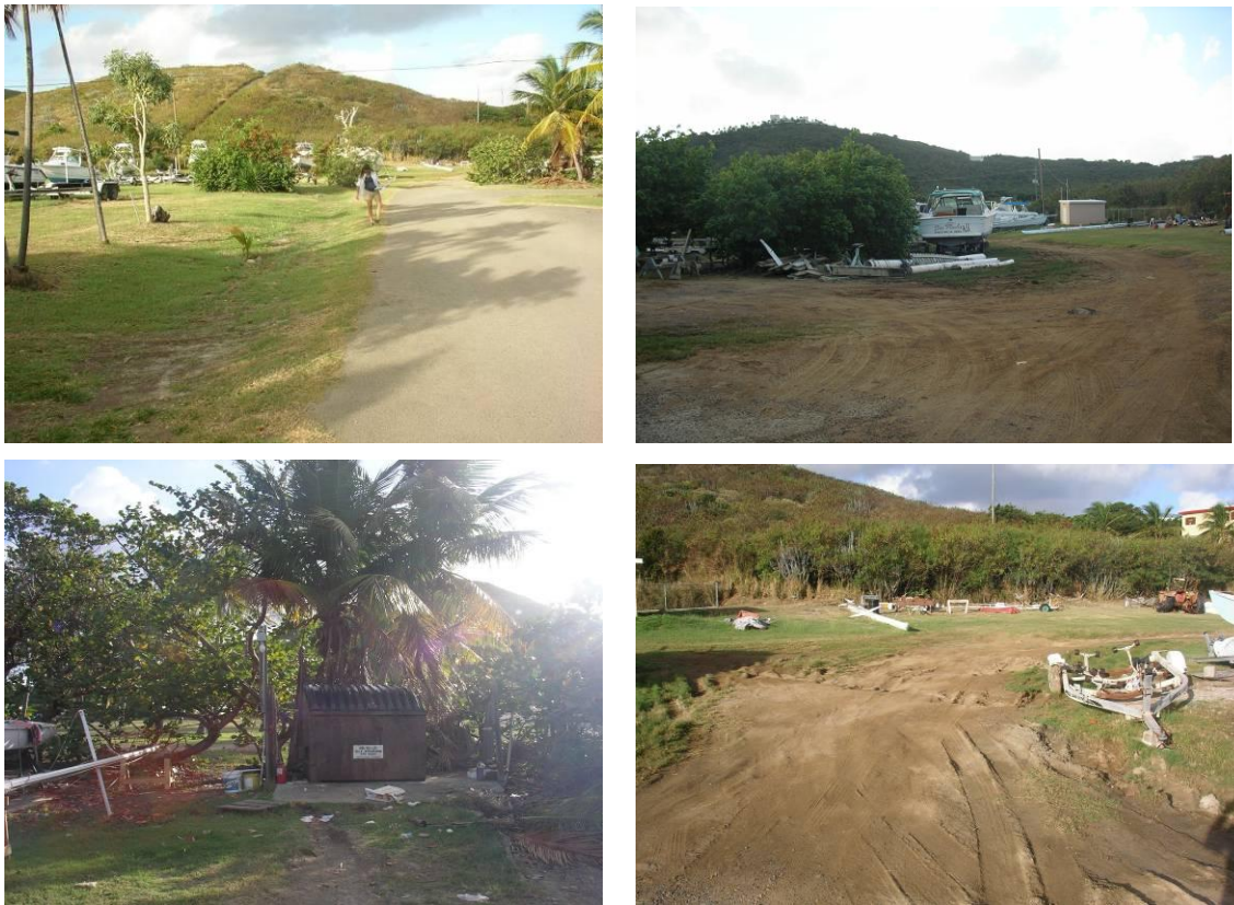
Figure 5.4. Drainage from a large portion of the watershed comes through this swale (top left); Stormwater flows overland across unvegetated/muddy boat storage/parking areas (top right and bottom photos).
