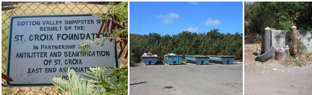
Figure 4.8. The rebuilt dumpster site is an important resource for the community (left). However, the dumpsters are uncovered, overflowing, and located directly adjacent to a gut (middle). Potentially hazardous materials are left in this area (right).
