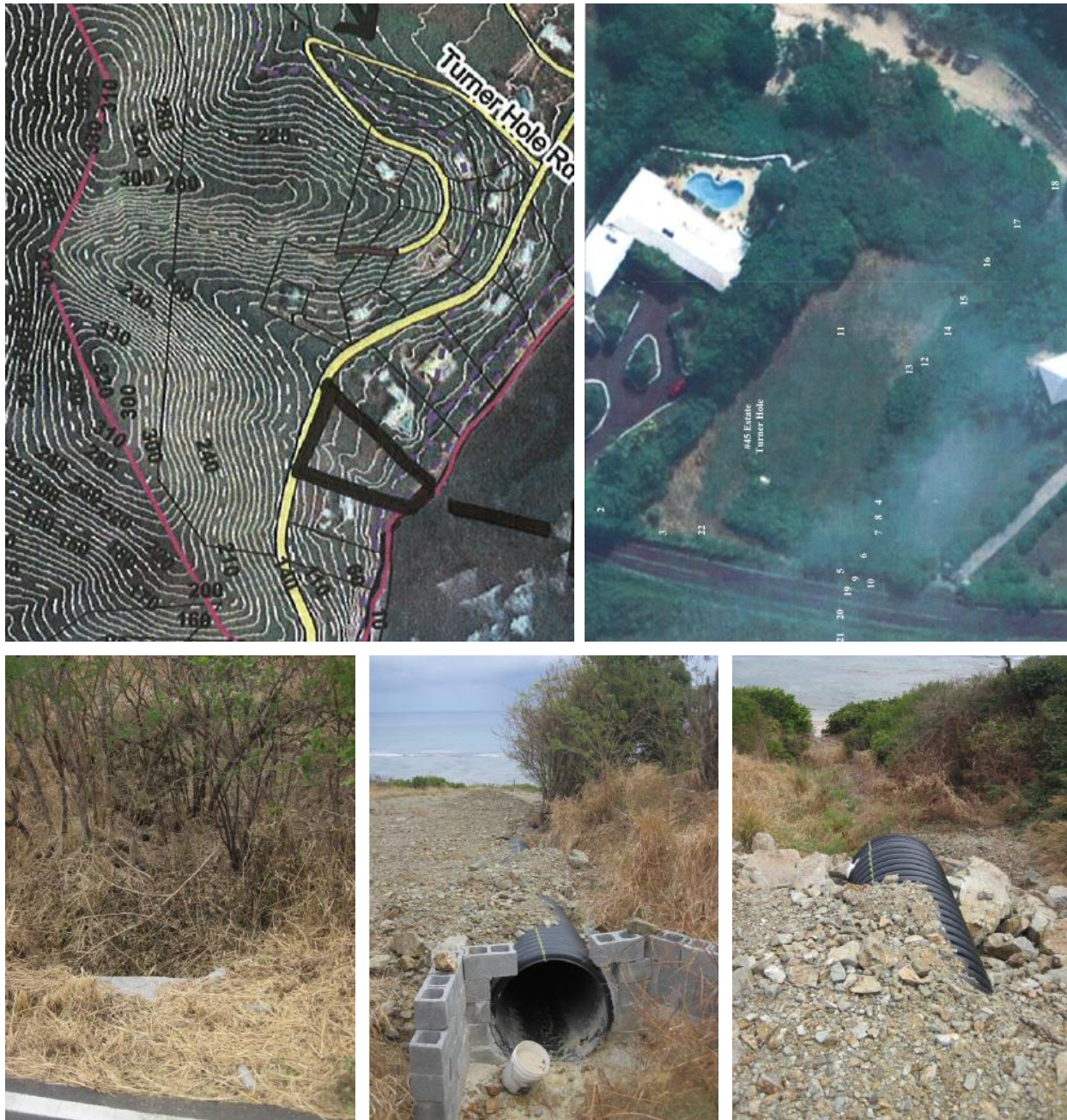
Figure 6.9. (From top left to bottom right) Parcel location; aerial photo of site with location along channel/culvert where photos were taken by EEMP staff; looking at gut above road crossing; new culvert inlet on property, and culvert discharge to bay (photos from EEMP staff on March 14, 2011).
