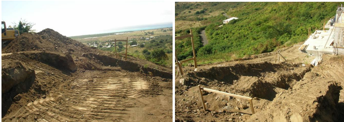
Figure 8.13. Slope clearing at residential construction site in Marienhoj.
