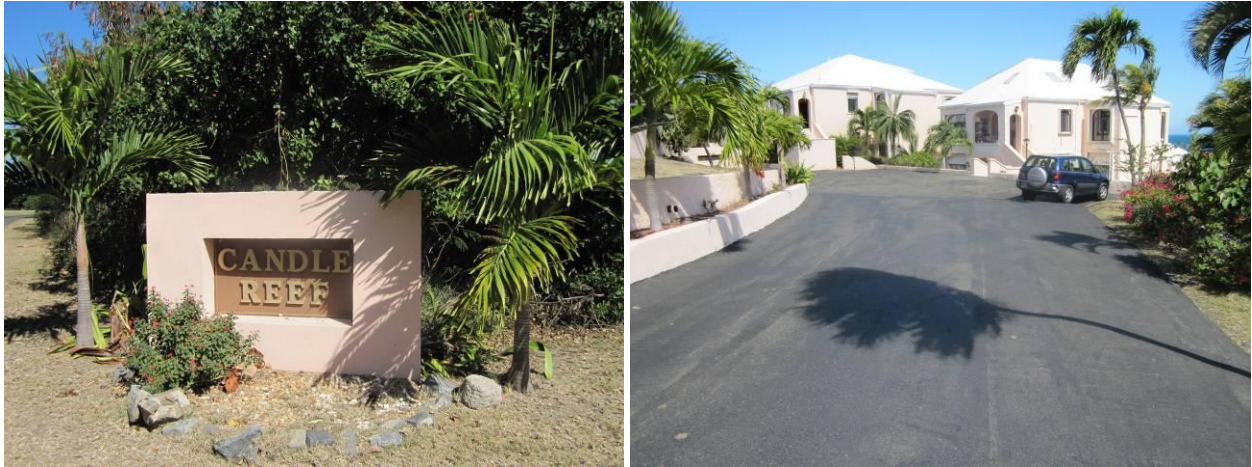
Figure 4.45. Entrance to Candle Reef condominium complex (left) and paved road leading to condominium units (right).
