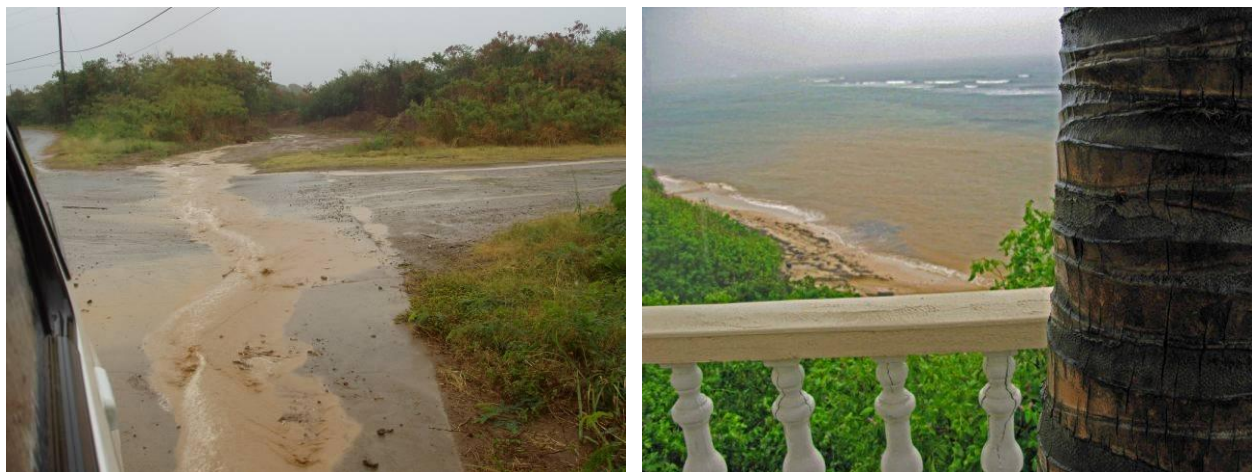
Figure 1.3. Sediment-laden runoff from unpaved roads in Cotton Valley conveyed in concrete swale (left, photo courtesy of Zandy Hillis-Starr). Uncontrolled runoff resulting in sediment plume in Grapetree Bay during heavy rains in July 2010 (right) (photo courtesy of Kathy LaGrange/Dave Rivers).
