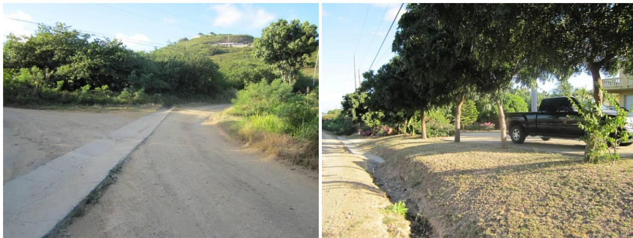
Figure 4.38. Concrete swale installed along dirt road in Hope and Carton Hill neighborhood (left) and erosion along dirt road where a paved swale ends (right).
