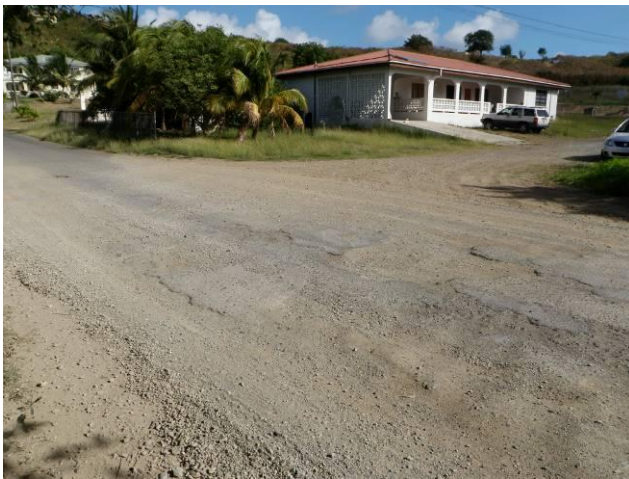
Figure 8.2. Unnamed, unpaved road (top photos) draining to South Shore Rd. deposits sediment across South Shore Rd. into vegetated area and is contributing to road surface degradation (bottom photos).
