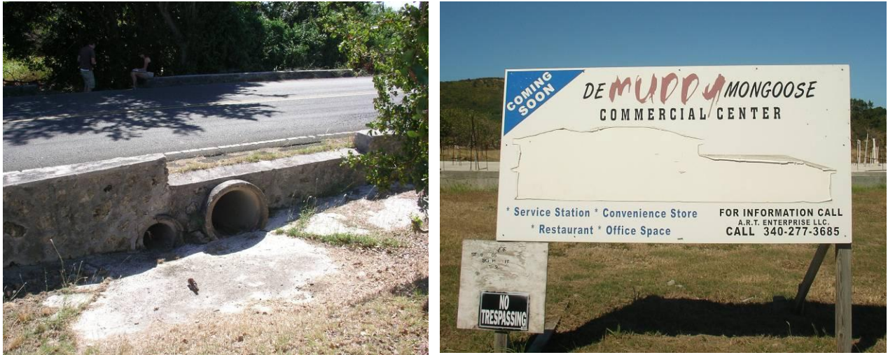
Figure 8.6. Culvert near Muddy Mongoose proposed development.
