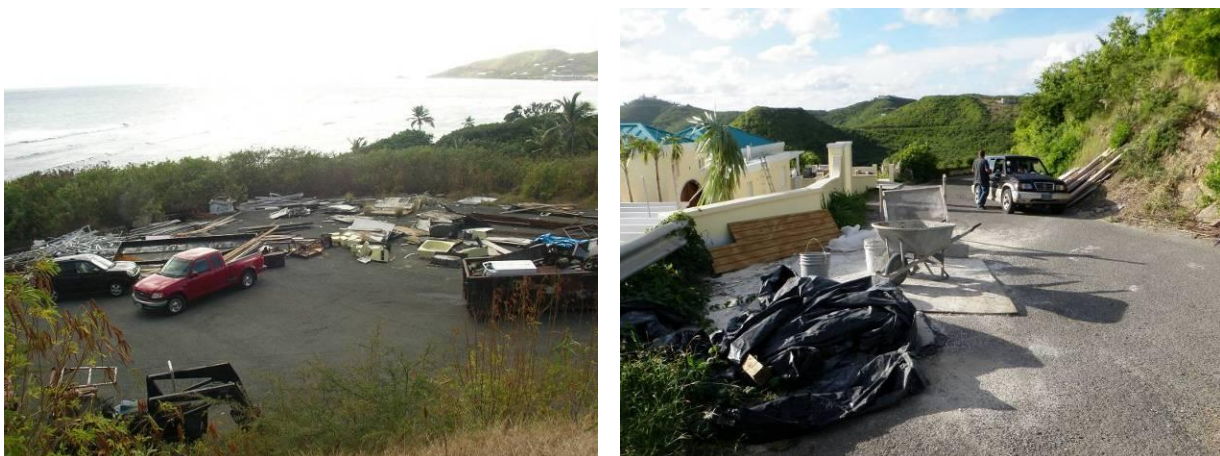
Figure 6.5. Parking lot and construction materials/debris storage at the Grapetree Bay Hotel (left). Material storage and staging at small residential construction site in Turner Hole (right).
