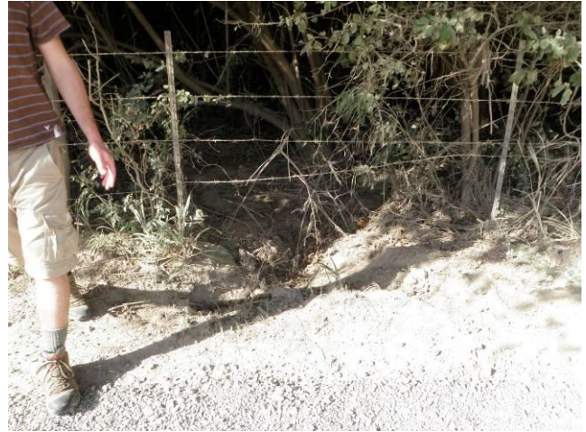
Figure 8.2. Unnamed, unpaved road (top photos) draining to South Shore Rd. deposits sediment across South Shore Rd. into vegetated area and is contributing to road surface degradation (bottom photos).
