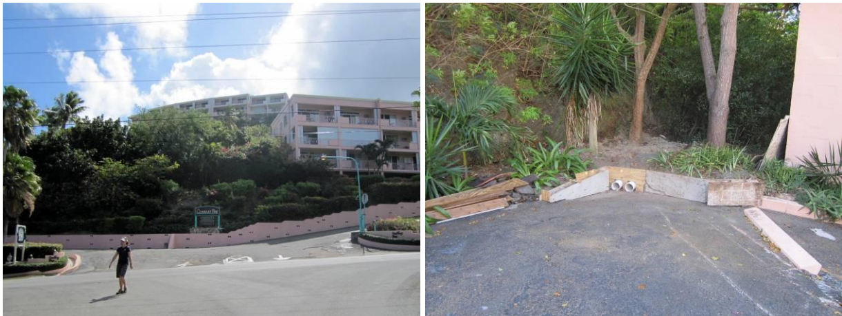
Figure 4.17. The majority of uncontrolled stormwater from the site flows down to the entrance and then along the edge of East End Rd. (left). This is an area in the southwest corner of the upper parking area where water would puddle after rain events. Small PVC pipes have recently been added to drain this area, creating an ideal location for a retrofit BMP (right).
