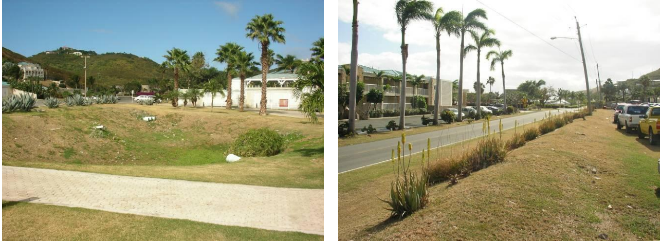
Figure 6.4. Detention basin at Divi Carina Bay Hotel & Resort (left). View of Divi Hotel parking areas along South Shore Rd and potential area for a rain garden/swale (right).
