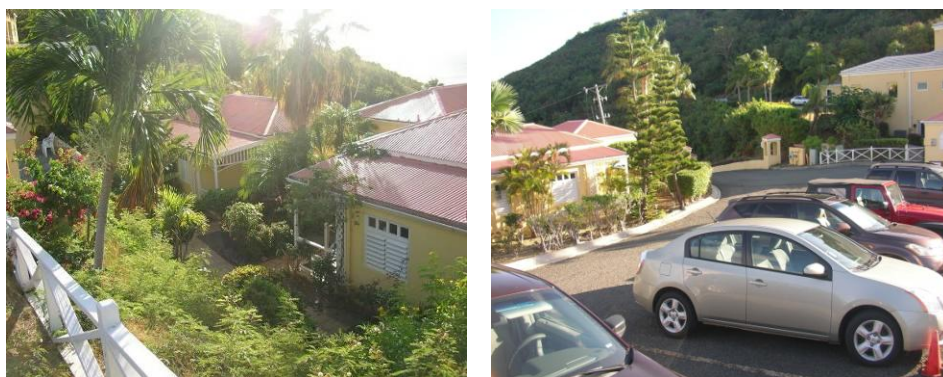
Figure 6.10. Condominium units and portion of parking area at Villa Madeline.
