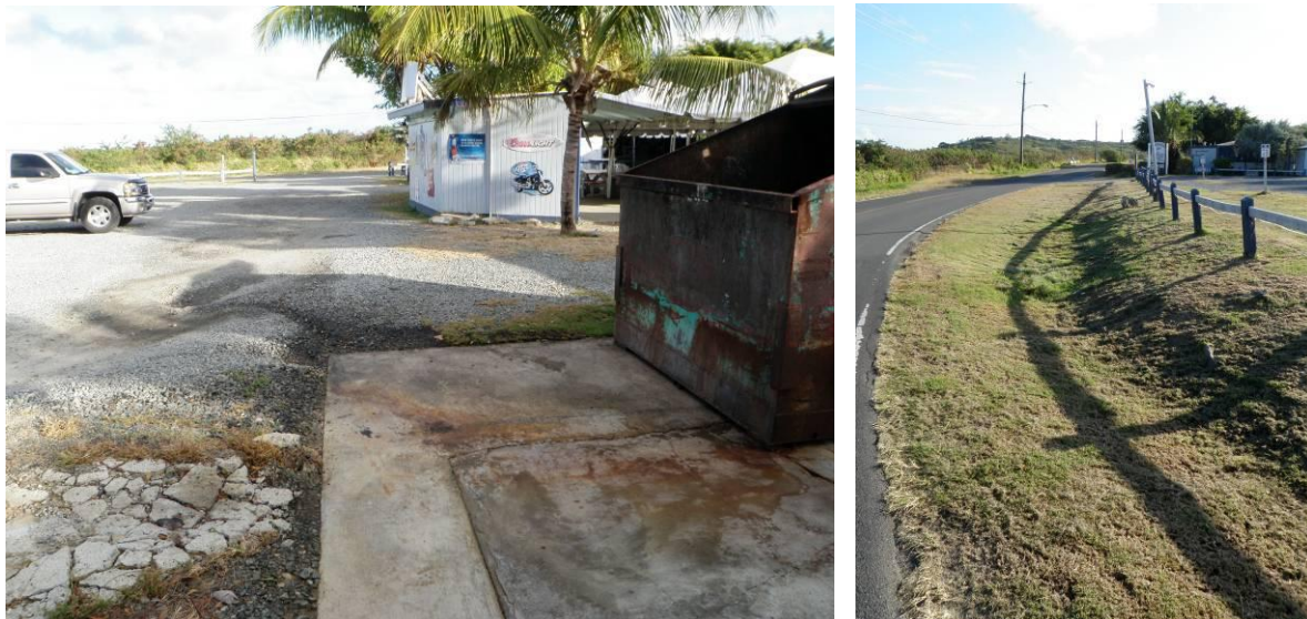
Figure 3.9. Evidence of dumpster juice in stormwater runoff (left); location for swale enhancement to increase water quality treatment.
