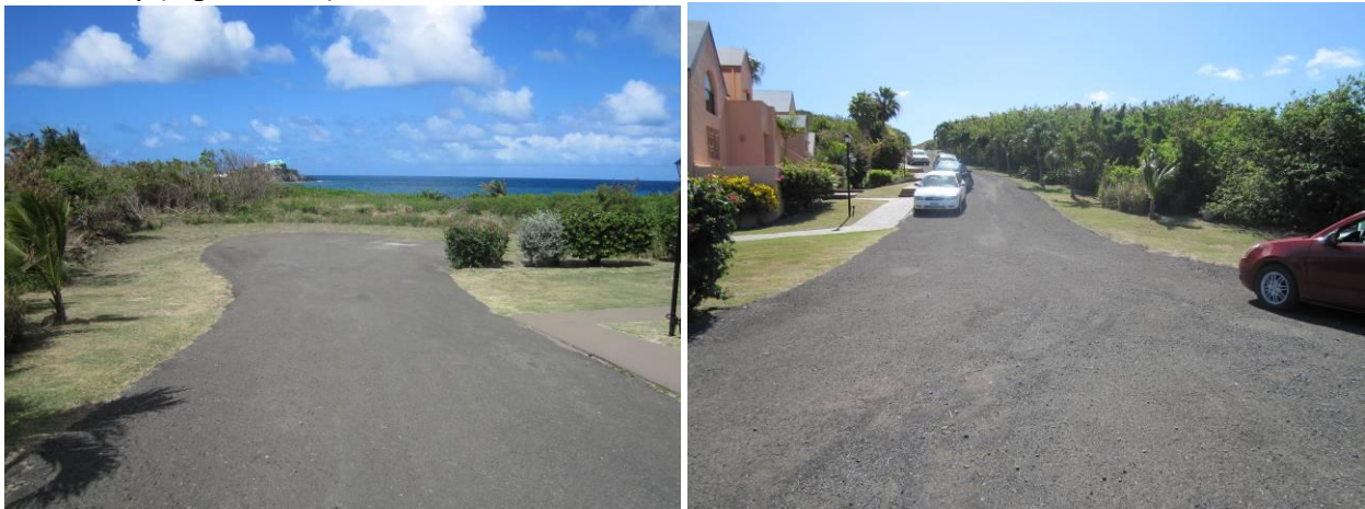
Figure 4.23. Prune Bay can be seen just beyond this large cul-de-sac near Candle Reef Condos II (left) and the drainage area to the cul-de-sac, consisting of roadway, parking areas, and walkways (right).
