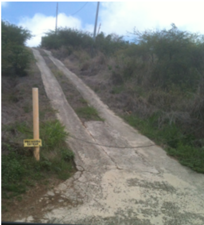
Figure 8. Example of a road on a steep slope that seemed to have minimal impact - two track drive - minimal impervious cover and crowned in the middle. This is a potential BMP for steep high use areas.
