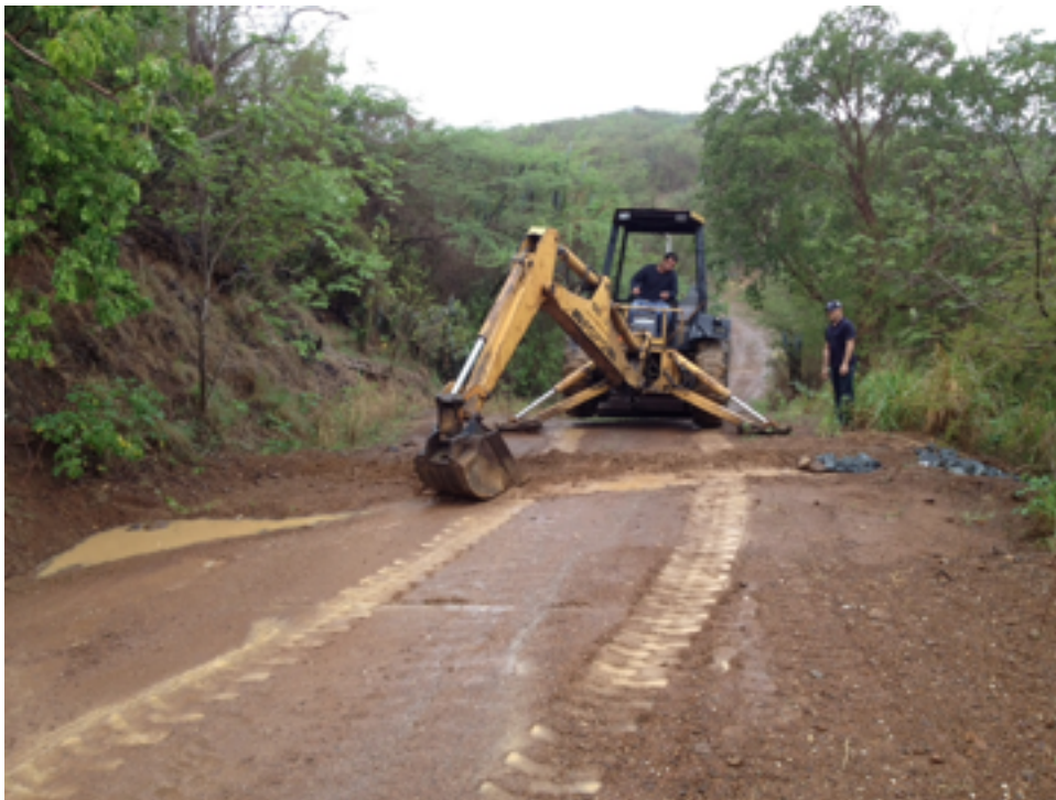
Figure 3. Illustrates the construction of a cross swale and outlet protection
