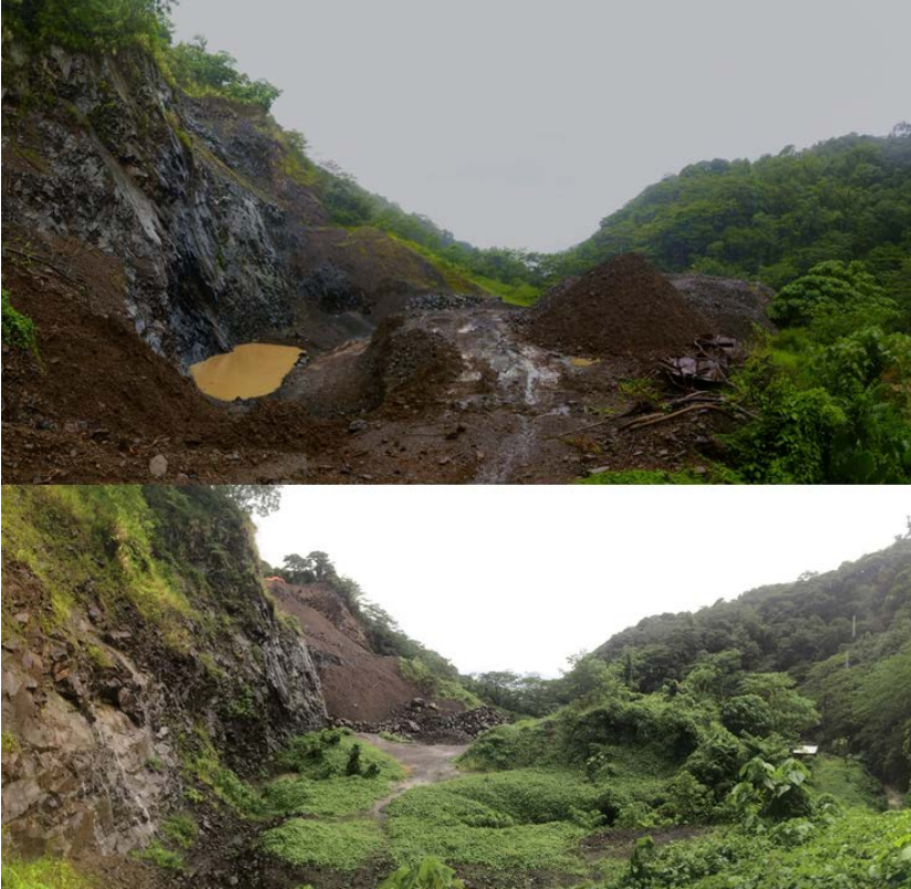
Figure 5. Pictures of the Excavation Platform before (2012, top) and after (2014, bottom) vegetation overgrowth of overburden piles. The groundwater seep is evident in the muddy puddle in the top picture. The groundwater diversion routed this flow to the right in the picture, into the stream before it could erode the Platform surfaces. Pictures taken by Alex Messina.
