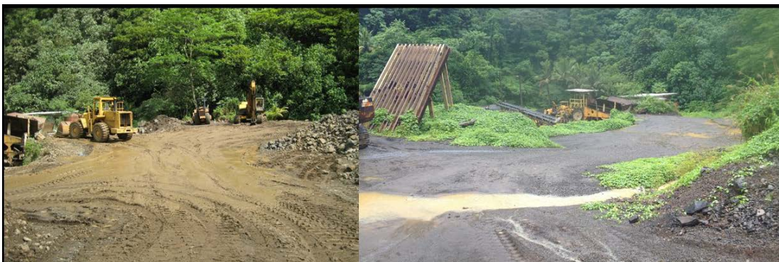
Figure 4. Pictures of the Upper Operational Area before (left) and after (right) covering road surfaces in gravel. Pictures taken by Alex Messina
